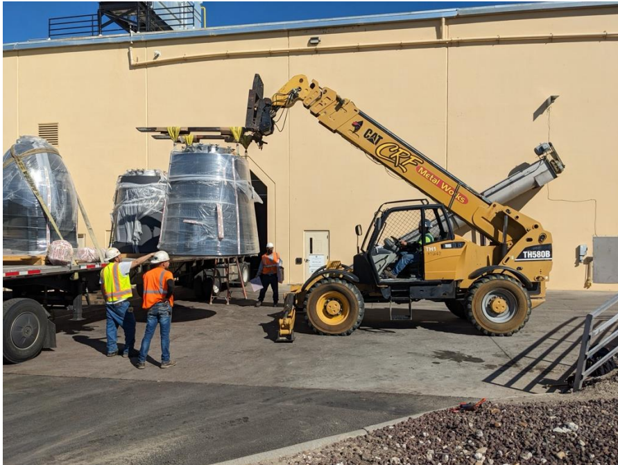
Lifting from Above with Rigging Material and Telehandler
